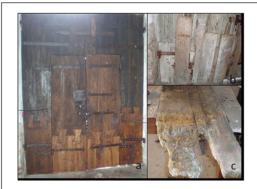
Figure 2. (a) Vertical board assembly in the inner side, after the intervention. (b) Detail of the conservation state before the intervention and (c) decayed boards in the lower zone, inner side, during restoration.
