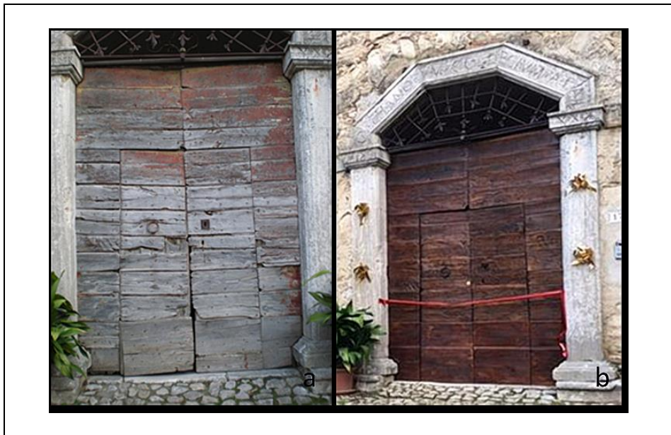
Figure 1. The door in the ex-Abbey of Saint Secondo: (a) before and (b) after the intervention. A smaller door is opened within the main one.
